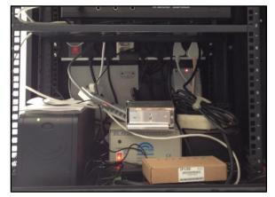
Figure 7: Example of Poorly Organised Security Equipment Cabinet
